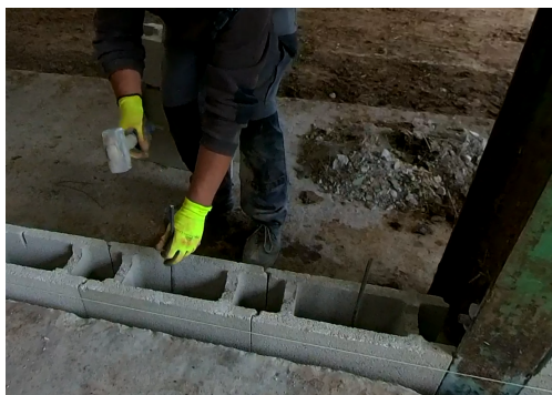
Installation of metal reinforcement bars
